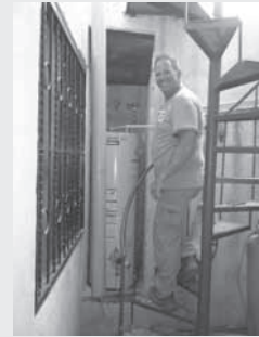
Dave installs the water heater.
